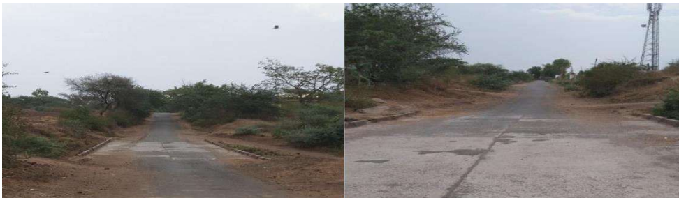
Figure 7: High Slope Road Connecting the Bridge
