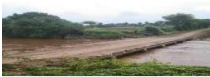
Figure 1: High Level Causeway at Naved-Darapur Road
