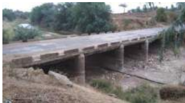
Figure 9: Lack of Lighting and Safety Signage
